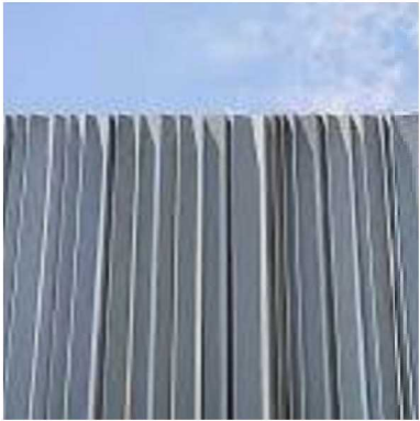
1. SUN SHADES MATERIAL: PROFILED METAL FINISH: SATIN COLOUR: SHADES OF GREY
